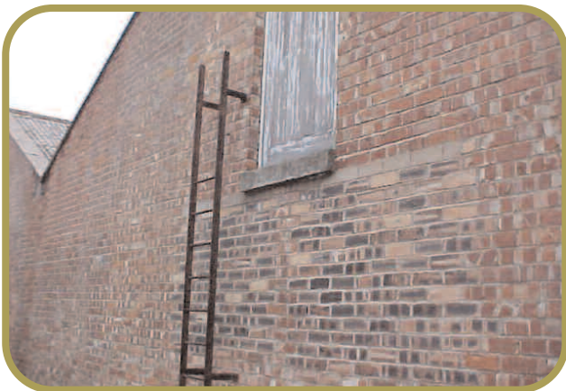
External fire escape, very difficult to reach from inside loft and no warning signage on the inside of this door to inform of drop
